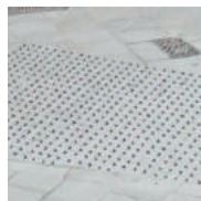
Conservation tactile paving
