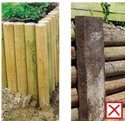
Timber log retaining wall to the public realm will not be acceptable.
